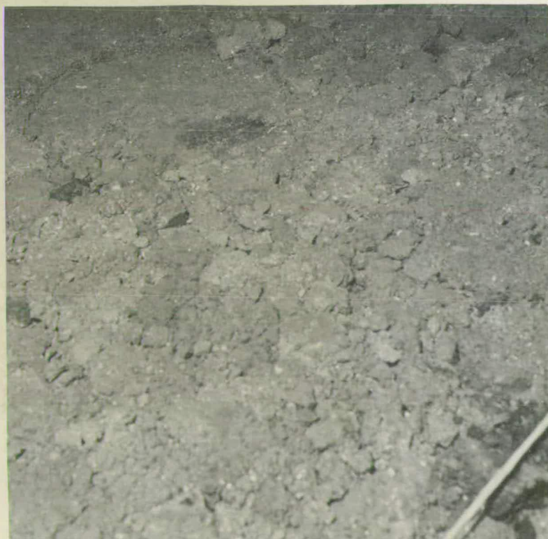
MARK ON ROAD BASE AFTER C.B.R. TEST
