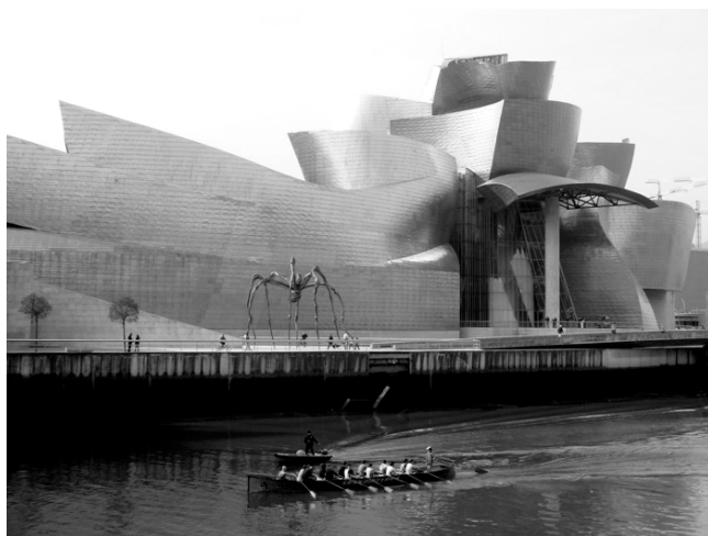
Figure 1.3: Frank O. Gehry: The Bilbao Guggenheim Museum, Bilbao, Spain, 1997. Source: the author.
