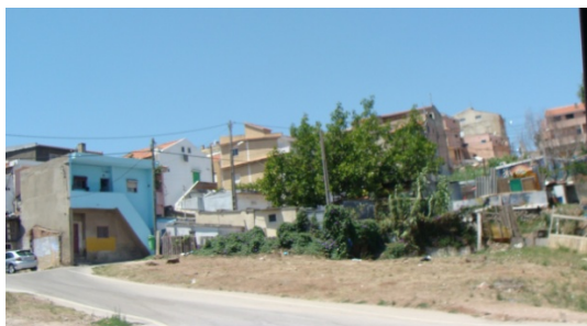
a) Cova da Moura (illegal construction)
