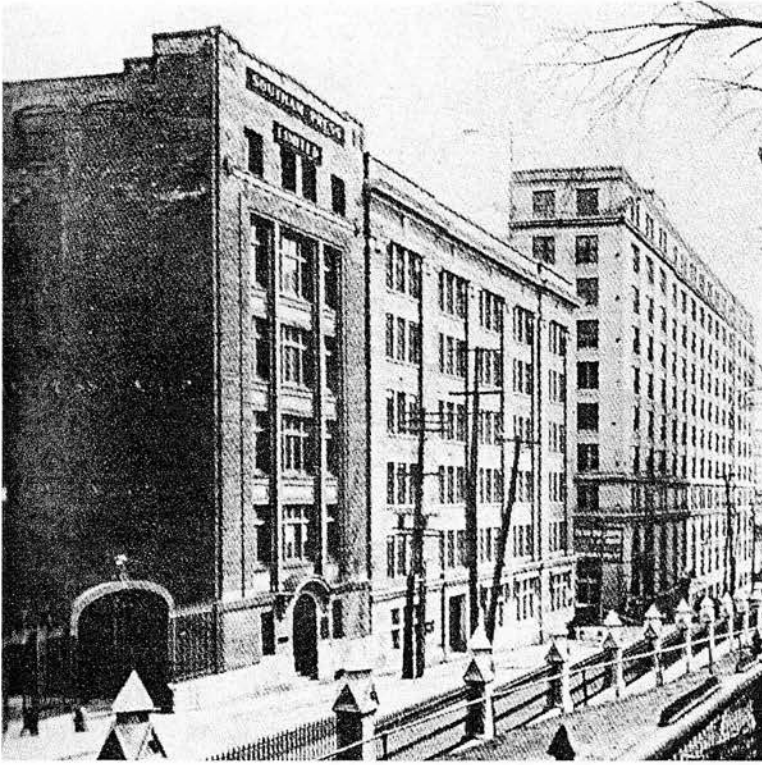
167. Brown and Vallance, Southam Building to left of picture (1913) (Gournay and Vanlaethem, Montreal Metropolis )
