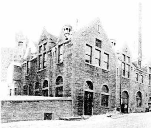
122. Taylor, Power Plant, Royal Victoria Hospital, Montreal (1900) (McGill University Archives)
