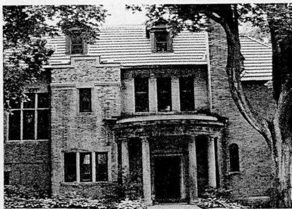
85a. Findlay, House for R. Macaulay, Avenue Cedar, Westmount (1911) (Photograph, Kinnear)
