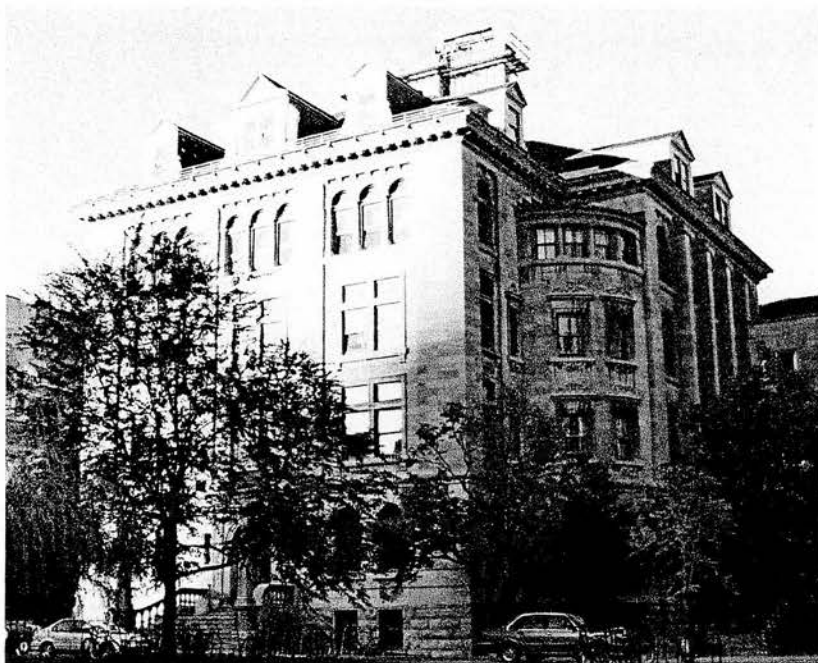
63. Taylor, McGill University, Macdonald Chemistry and Mining Building (1896) (Photograph, Kinnear)
