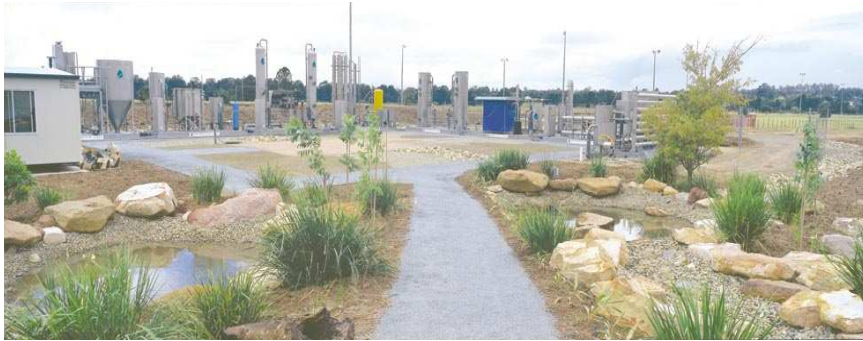
Figure 1: View of the Advanced Water Recycling Demonstration Plant
