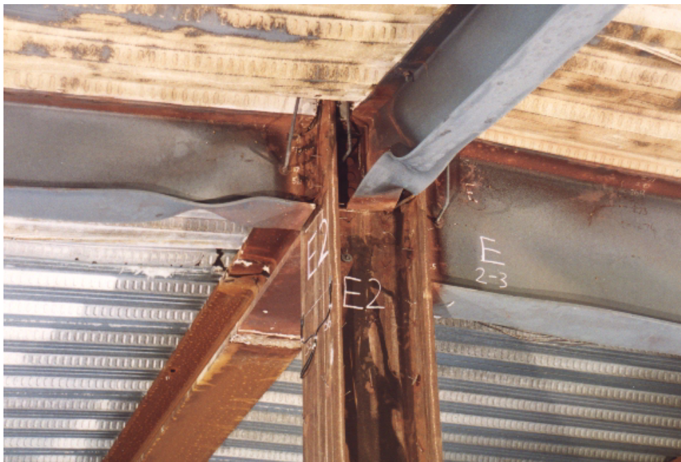
Figure 4.6: Local buckling of beams in British Steel Test 3: Corner test
