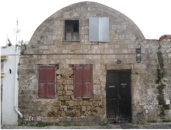
Figure 61: The main facade on Kisthiniou Street
