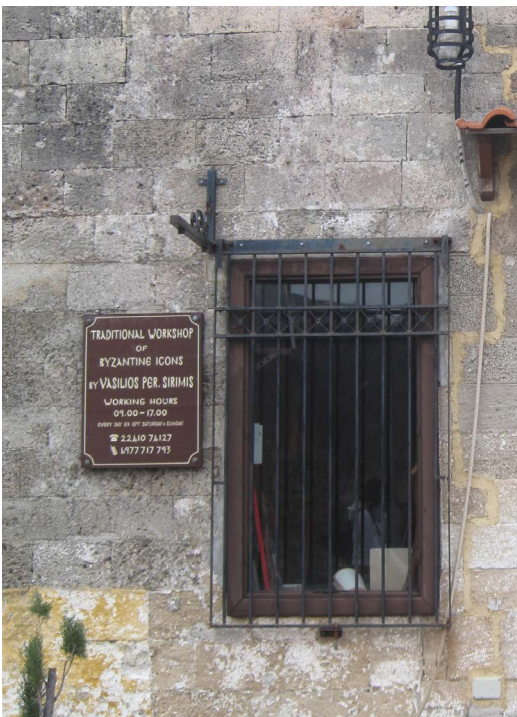
Figure 58: Replacement with new window frames
