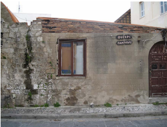
Figure 62: The restoration of the right part of the building with new sandstones
