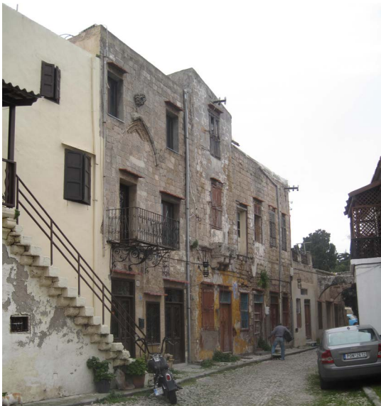
Figure 47: The street facade of the complex
