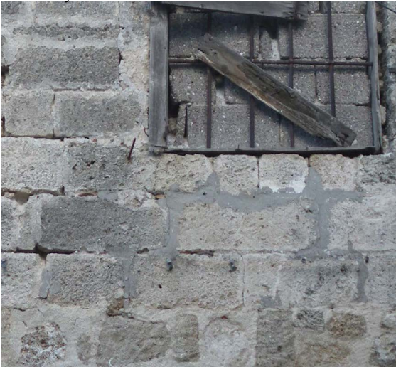
Figure 43: The impermeable cement mortar from the Italians
