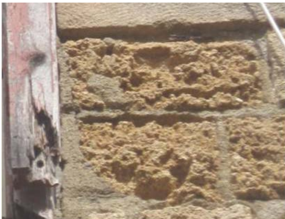
Figure 44: Honeycombing pattern due to different properties of stones
