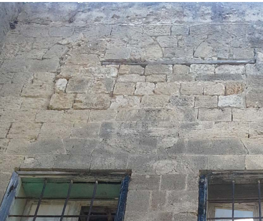
Figure 73: Blocked arched windows
