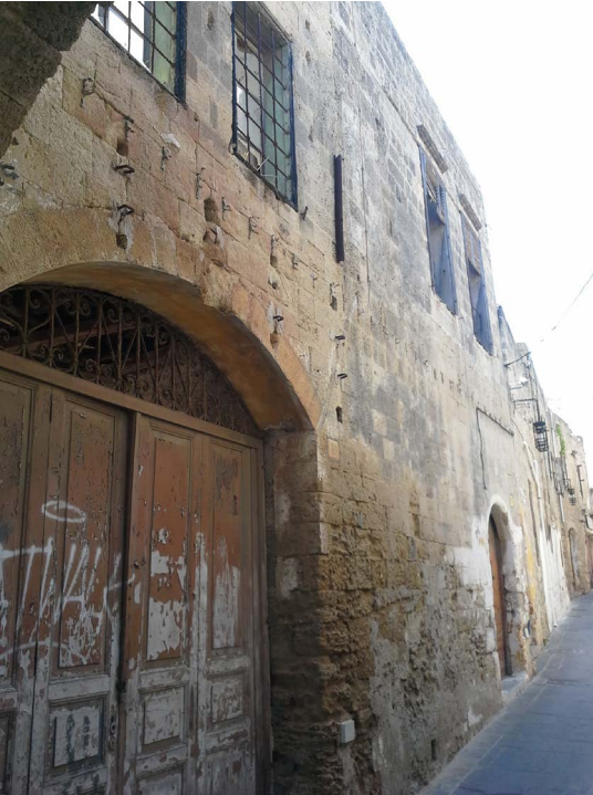
Figure 70: The main facade
