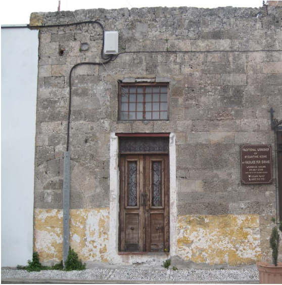
Figure 54: The ground floor of the building facing the street
