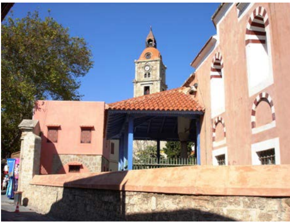
Figure 25: Kourasani mortar used as a coating material on the Suleyman mosque in Rhodes
