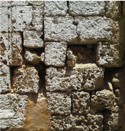
Figure 93: Honeycombing pattern
