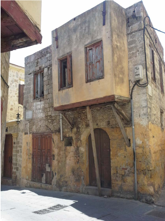
Figure 83: The building in the corner of the street and the enclosed sachnisi
