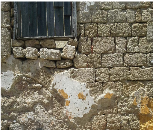
Figure 94: Case hardening of sandstone
