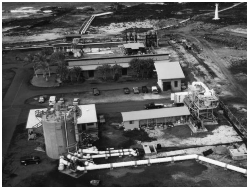
Figure 1.15: Land based view of the 210 kW OTEC Experimental Plant, Hawaii ( www.rise.org.au/info/Tech/otec/image007.jpg )
