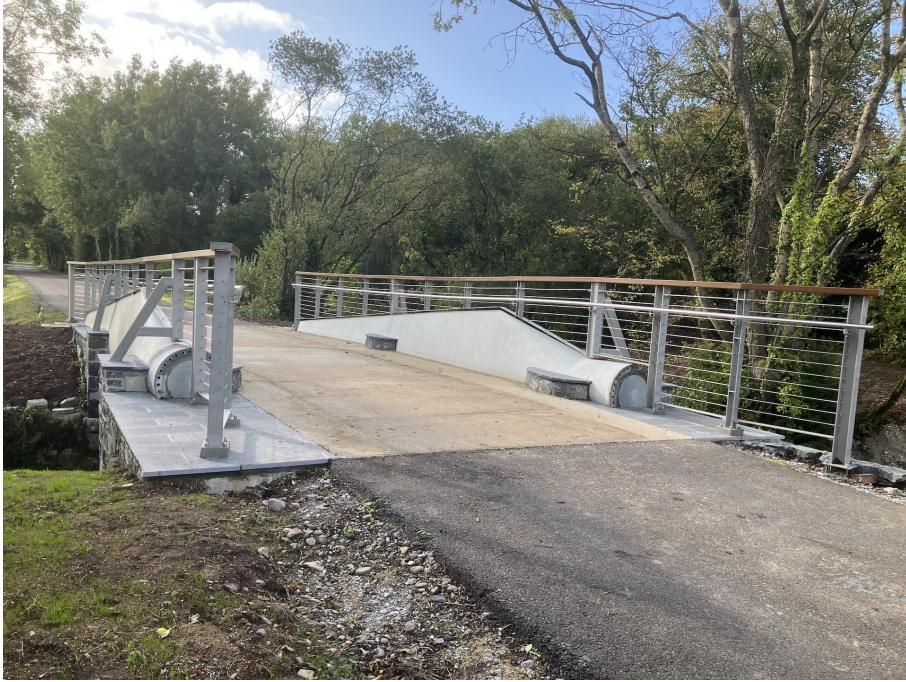
Figure 2.2: A pedestrian bridge installed by BladeBridge [17] in 2022. Used wind turbine blades provide structural support. Image reproduced from [17].
