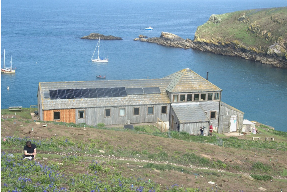
Figure 5. The “North Haven” colony of Manx shearwater, and the building accommodating the warden, most researchers and the Skomer library (06.05.2023)
