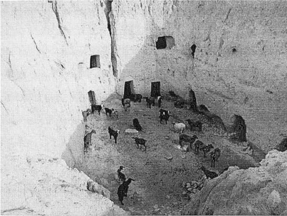
Fig. 4.1 In the absence of building material in this arid corner of Tunisia, early settlers dug into the soft earth to make living space that was warm in winter and cool in summer. But the government is keen to resettle people in modern homes on the surface, which is far from their environmental needs.
