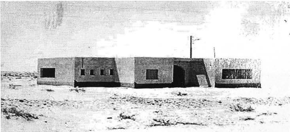
Fig. 11.8 Youth centre in El-Hasana (under construction)
