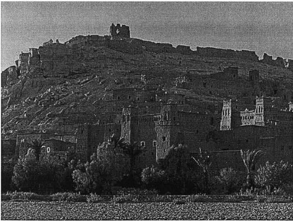
Fig. 2.6 Ancient Aït Benhaddou, Morocco, Impressive and elegant towers below but the neglected old fortification at the top of the hill is half reduced to ruin by rain and wind (Palin, M. 2002).
