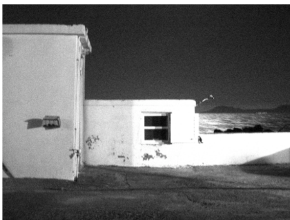
Figure 31: An extension to a small house
