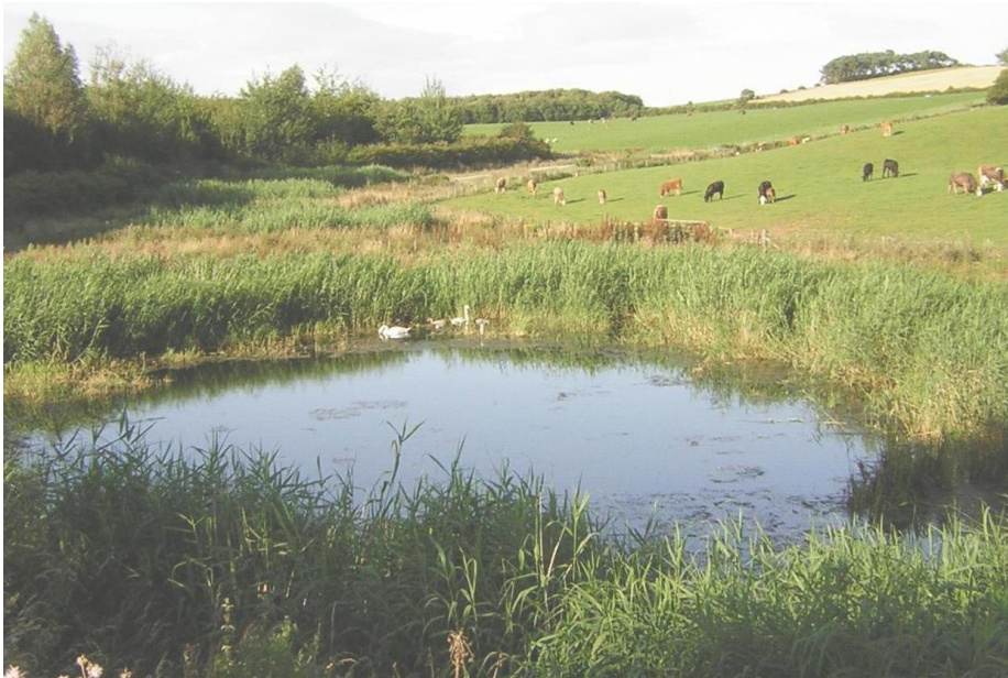
Figure 3.5 View of CFW2 (summer 2008), which comprises five ponds in series planted with P. australis around the edges. The last and largest pond is seen in the foreground. The CFW inlet is located in the background.
