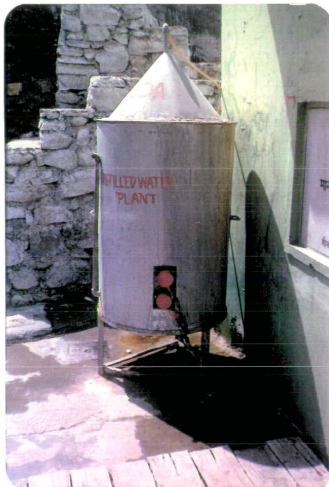
Photograph 5.9 Sahastradhara MHP project ELC ballast load - water distiller
