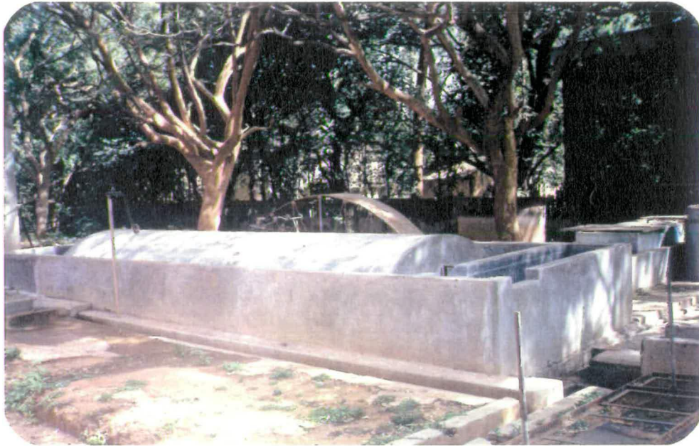
Photograph 4.1(b) Improved family biogasifier designed by ASTRA
