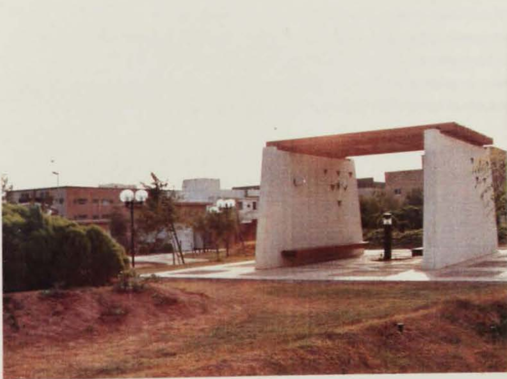
Fig 38: Lighting fixture replaced palm tree inside the shade structure.
