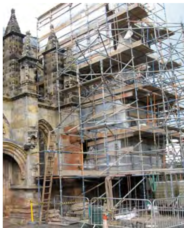
Figure 2.28 Pinnacles and buttress between bay S5-S6 during conservation treatment in June 2011.
