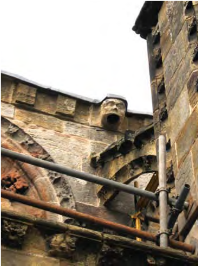
Figure 2.7 Detail of wall head showing grotesque above flying buttress.
