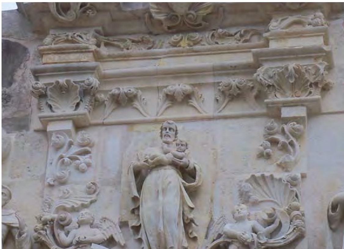
Figure 3.31 Upper portion of facade showing recarved 1949 cornice blocks and new limestone floral element to left of St. Joseph that replaced the inappropriate 1949 carving. Note how this new floral element is more consistent with the style and proportion of the existing original floral element to the right of St. Joseph. March 2011.
