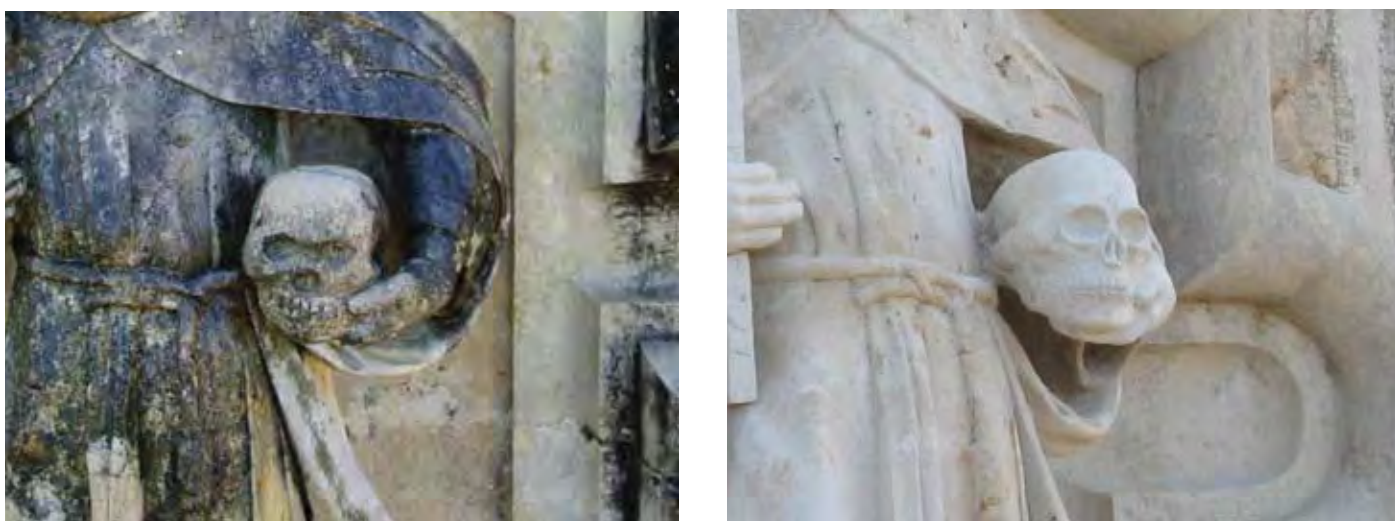
Figure 3.29 Replacement skull at St. Francis figure executed in cement in 1949 (left) before restoration in 2009 and after restoration (right) in 2011 with new carved stone indent secured to original stone behind with pins and grout.
