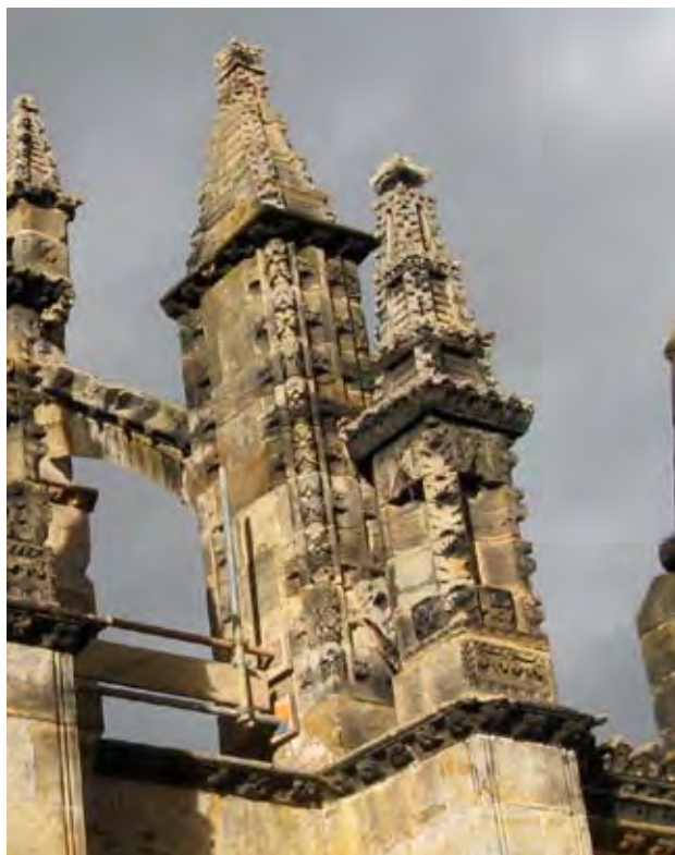
Figure 2.27 Pinnacles between bays S5-S6 before conservation treatment in 2010.
