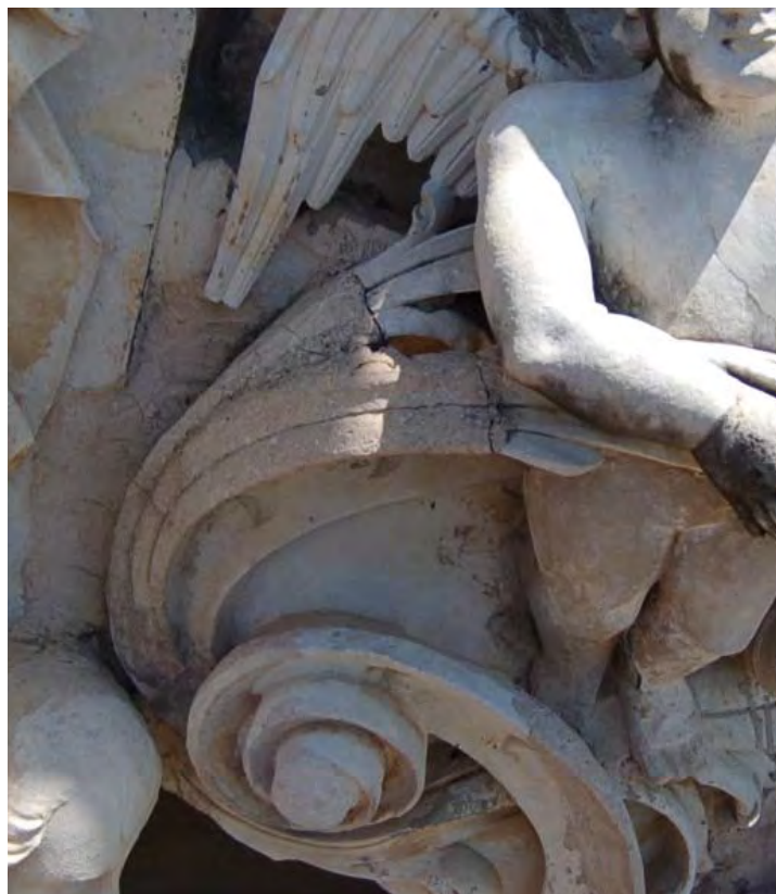
Figure 3.15 Detail of angel figure in zone G, showing cement patch of lost carved element adjacent to angel's proper right arm. February 2009.
