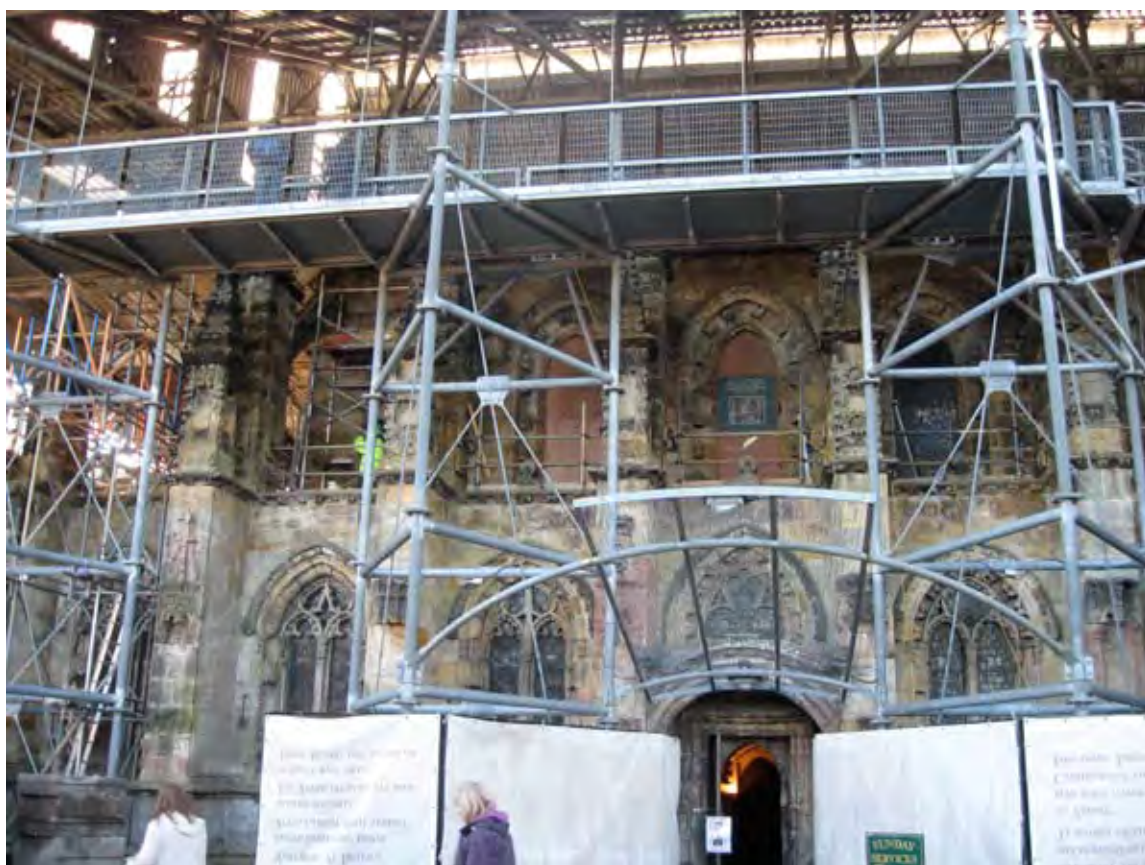
Figure 2.16 Rosslyn Chapel covered by temporary roof. December 2009.
