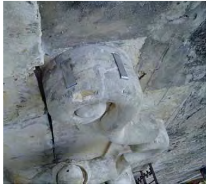
Figure 3.22 Cracked volute in zone H stabilized in Phase I with stainless steel cramps.
