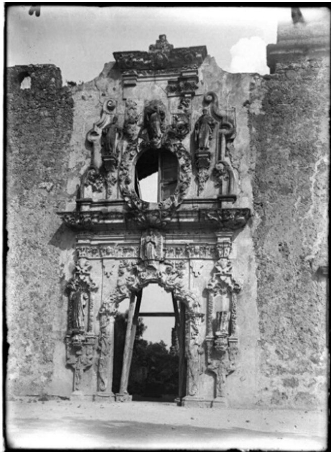
Figure 3.10 San Jose facade in 1917, showing bracing timbers supporting the facade wall.
