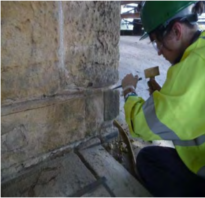
Figure 2.32 OPC mortar being removed from construction joints with hand tools. 2010.
