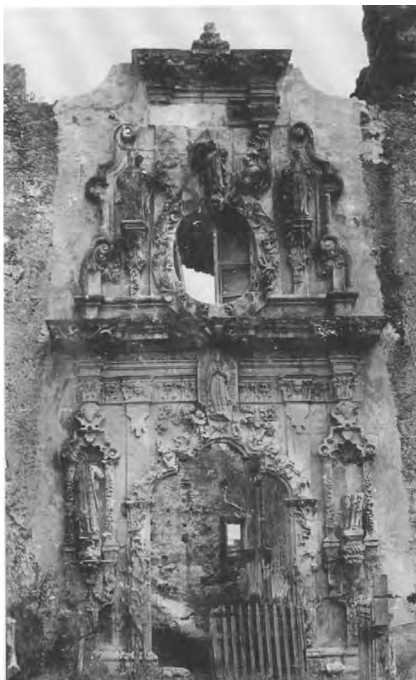
Figure 3.9 San Jose facade c.1890, showing loss of several sculptural elements and carved relief, as well as heavy dark staining on the stonework.
