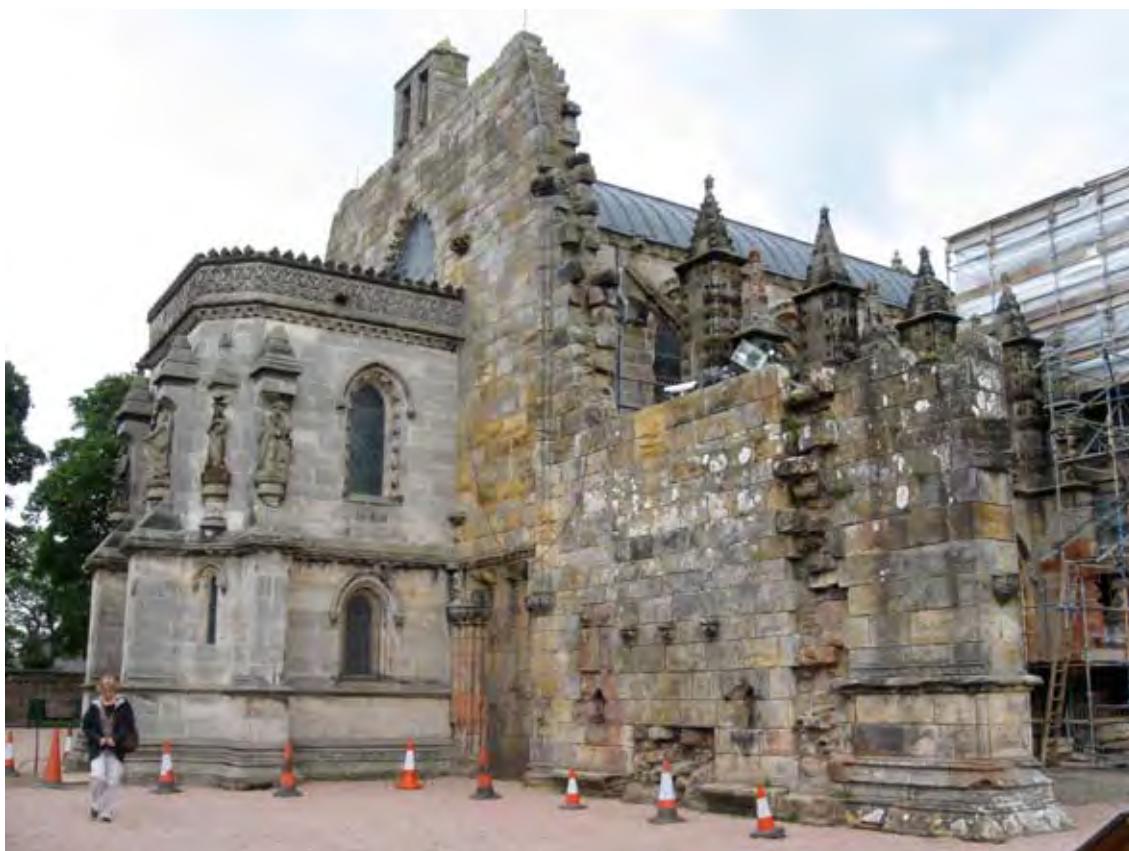
Figure 2.6 View of Rosslyn Chapel from southwest, showing transept walls and 1880 Kerr addition.
