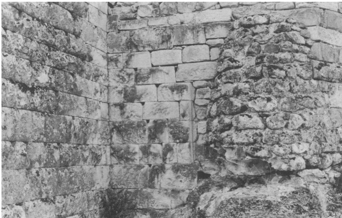
Fig. 10. Remnants of the fortification of Peium showing high-quality carved ashlar blocks. From Mitchell, 1974: 64.
