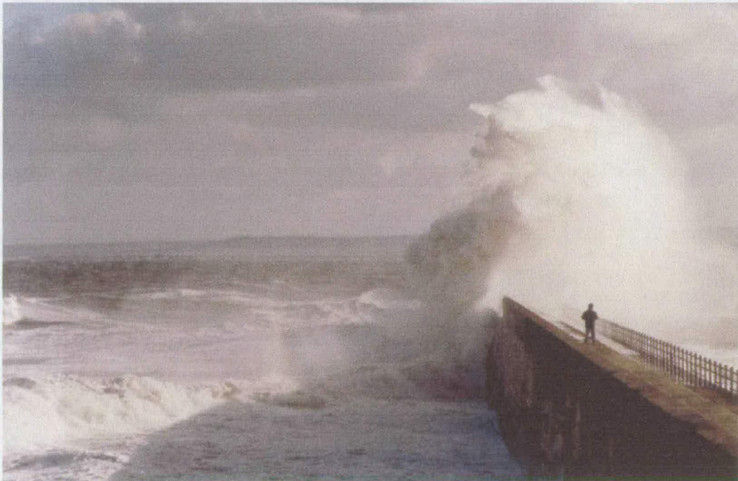
Figure 1: Oblique and Impulsive overtopping event at a plain vertical seawall (Hartlepool, courtesy George Motyka, HR Wallingford)
