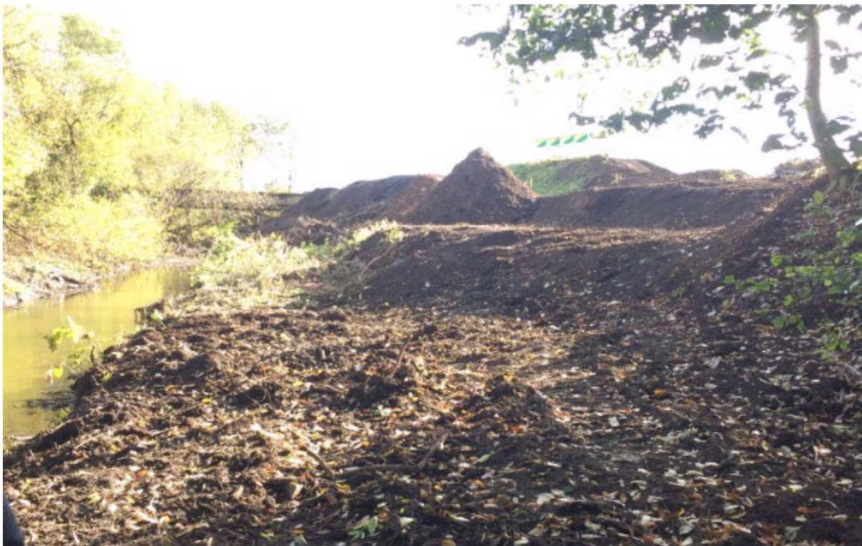
Figure 4-19: Earthworks showing disturbance of banking soil
