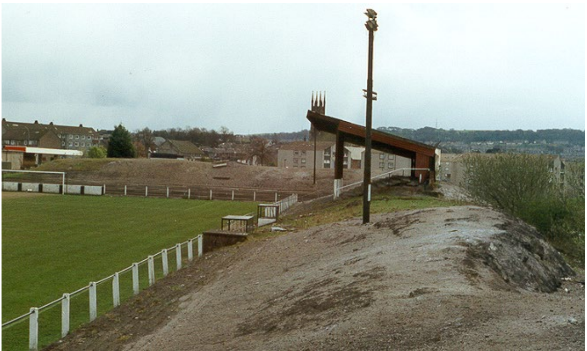
Figure 1-3: Photograph ca 2000 showing COPR used for terracing at Rutherglen Glencairn Junior Football Ground, south east Glasgow, Scotland (provided by Dr Margaret Graham, University of Edinburgh).
