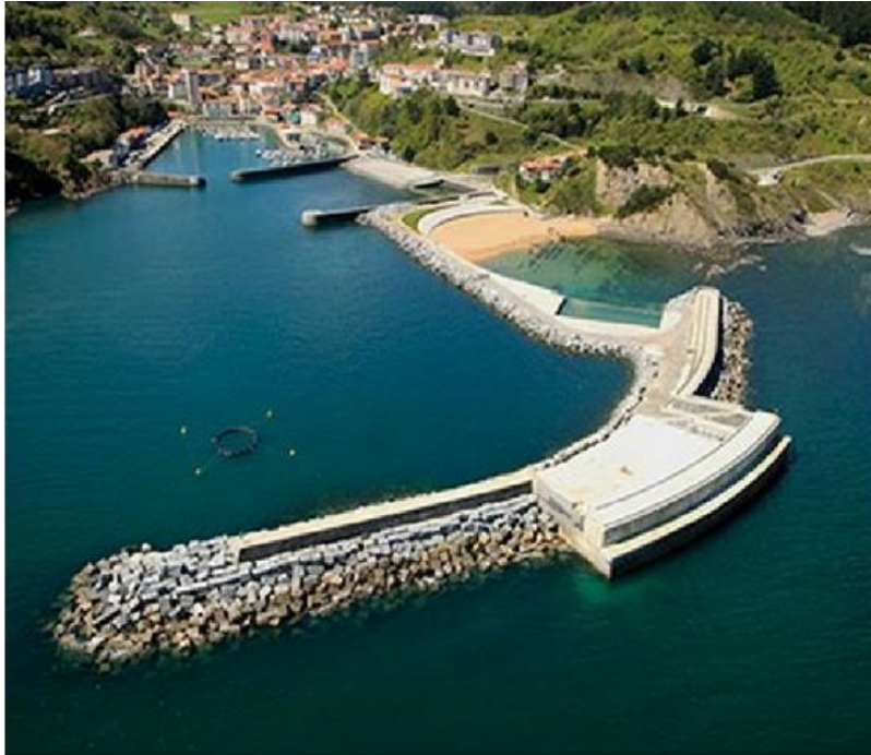
Figure 1-7: "OWC power plant at Mutriku" (Source: Garrido et al., 2015)
